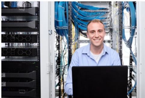
Reliable power for data centers
